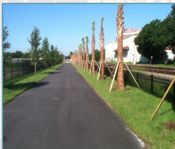
Trail with adjacent active rail line (Orlando, FL)
