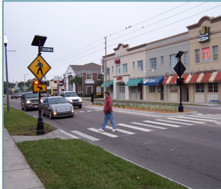
An example of an Enhanced Pedestrian Treatment with highly visible markings and a rectangular rapid flashing beacon (RRFB)
