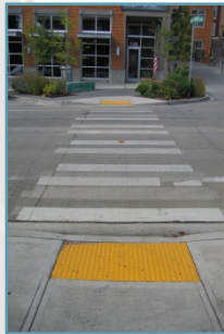
ADA pedestrian crossing (Bainbridge, WA)
