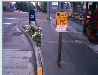
Loading zone & curb extension (Seattle, WA)
