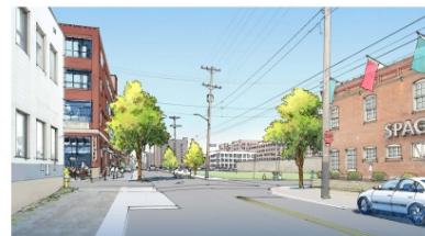
2. Renovation and improvement to existing buildings
